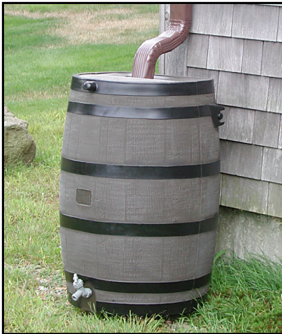
Typical rain barrel installation under downspout Photo: www.composters.com
