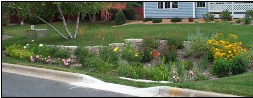
Example of a residential rain garden by the street. Note the cutout in the curb to allow water flow to and from the garden.
