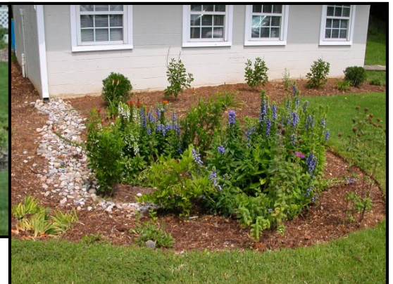
Downspout leading to a rain garden
